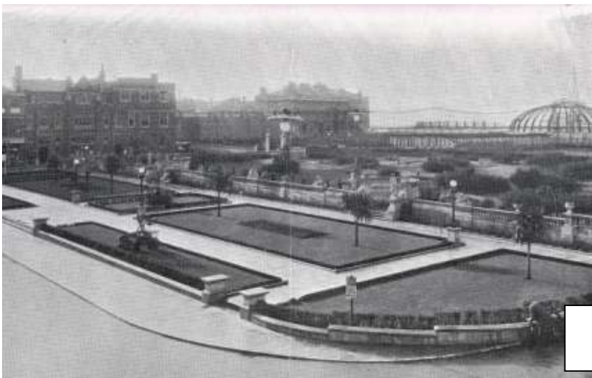
The pavilion under construction in 1925
