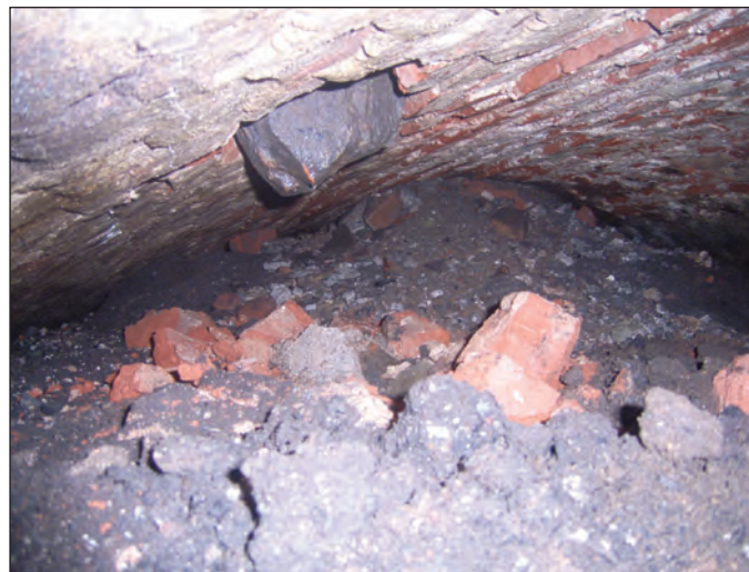
Plate 28 Internal view of cellar passage (122), showing brick structure of arched roof
