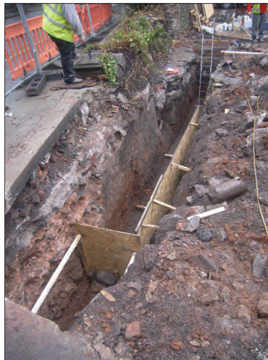
Plate 22 North-east facing elevation of wall foundation 129, exposed in a section of new foundation trench next to St Matthias Park (road)
