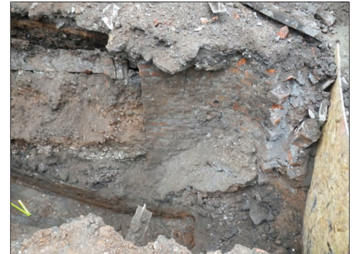
Plate 34 South-east facing elevation of foundation trench, showing brick-built ?access shaft into cellar passage, close to New Street frontage
