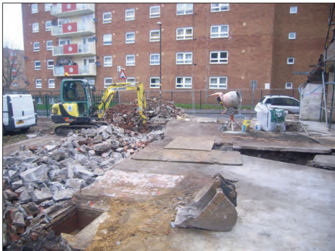
Plate 10 Breaking-up part of concrete floor slab (100), looking north towards New Street
