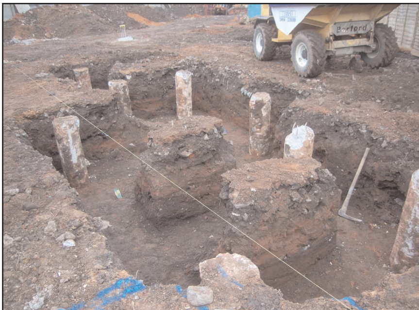
Plate 3 Adjoining ground beam slots as excavated in the south-west part of site (Flat 3 & cycle store) looking north, 0.5m scale
